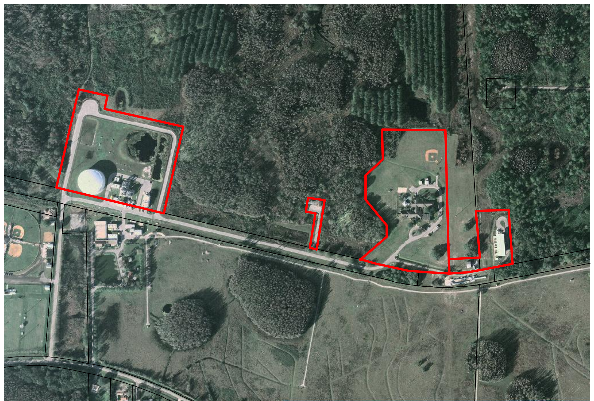
FIGURE 6- AERIAL HYDROGEN-SULFIDE FACILITY, ALCOHOL TREATMENT FACILITY, RADIO TOWER, INTERIM CHEMICAL FACILITY
